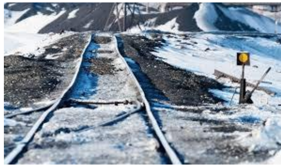
Svalbard: About 250 homes, traditionally built on wooden beams resting on permafrost, are to be demolished and housing relocated
